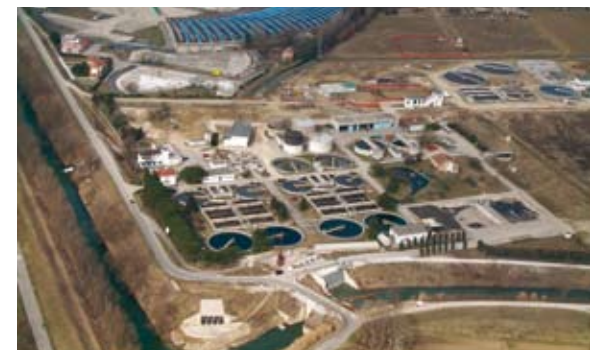
Il depuratore Ca' Nordio a Padova Padova's water treatment plant
