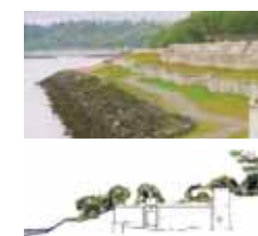
west point wastewater treatment plant, seattle, wa
