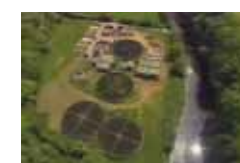
exeter wastewater treatment plant, uk
