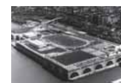
n. river wastewater treatment plant, ny
