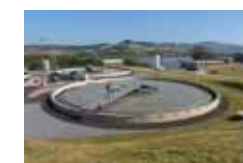
mechanical tertiary treatment
