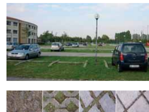
green parking lots with porous pavement
