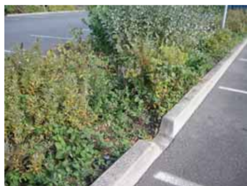
curb cuts define planting edges in parking lots and allow water to flow into bioretention areas
