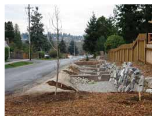
curbless street and bioswale water retention system
