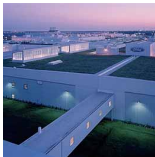
green roofs reduce stormwater runoff and moderate climate in buildings
