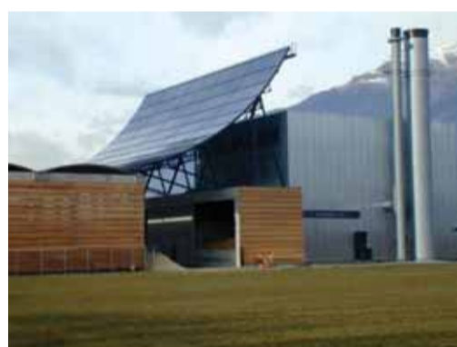
solar thermal collectors for hot water, heizhaus-lienz, germany
